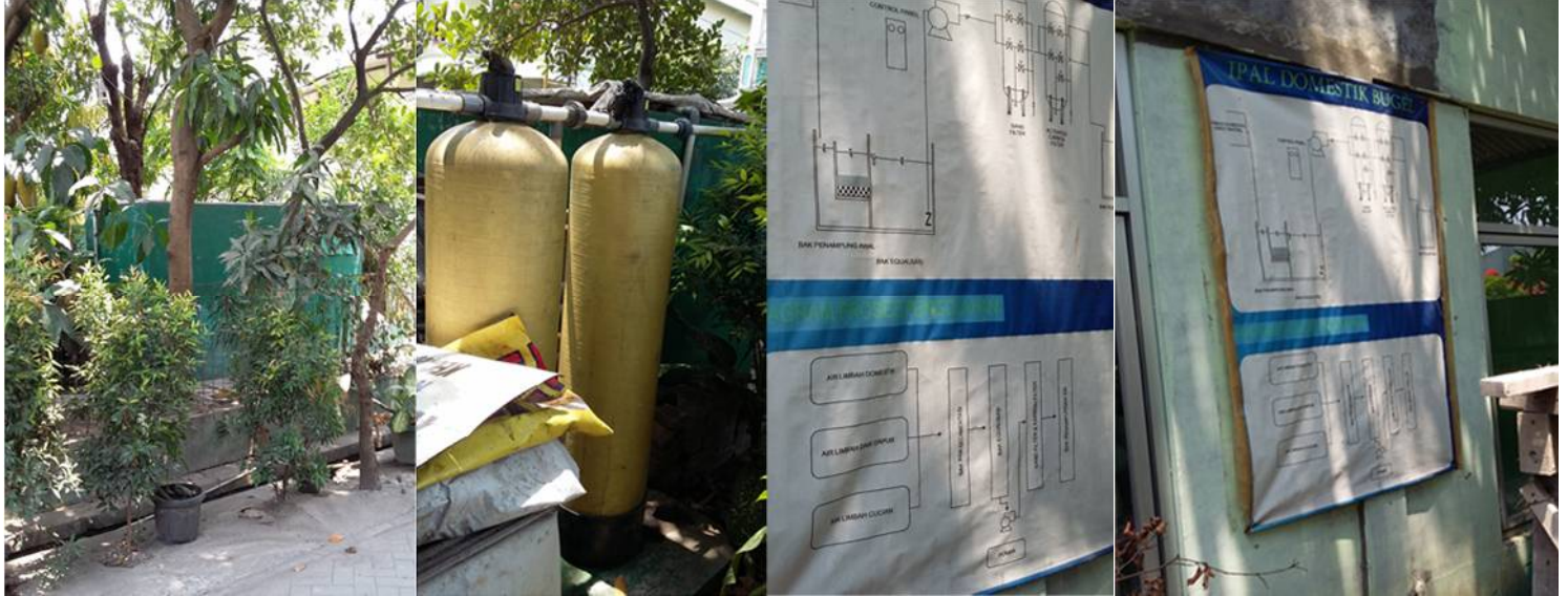
Communal wastewater treatment plant
