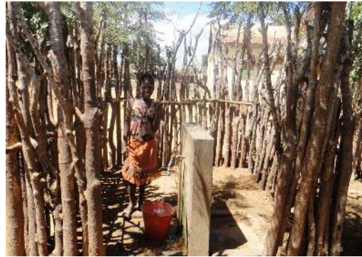
User fetching water from a fountain connected to a pumping water supply system
