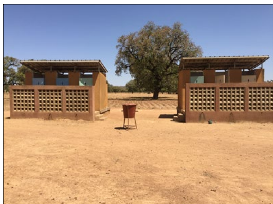
Gender-segregated school toilets at “Sho” in Koulikoro
