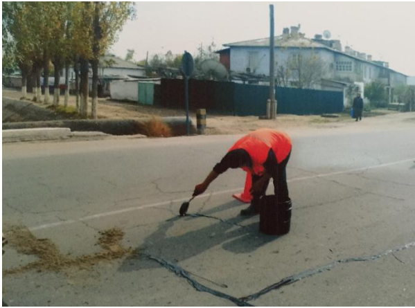
Repairing the cracks of the road surface by sealing (At the time of the ex-post evaluation)
