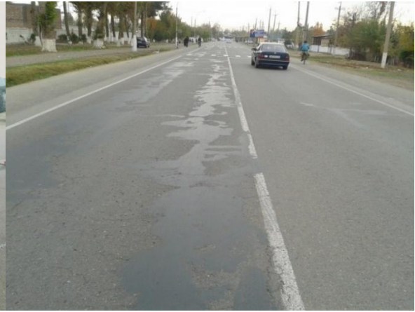
Road condition after repair (At the time of the ex-post evaluation)
