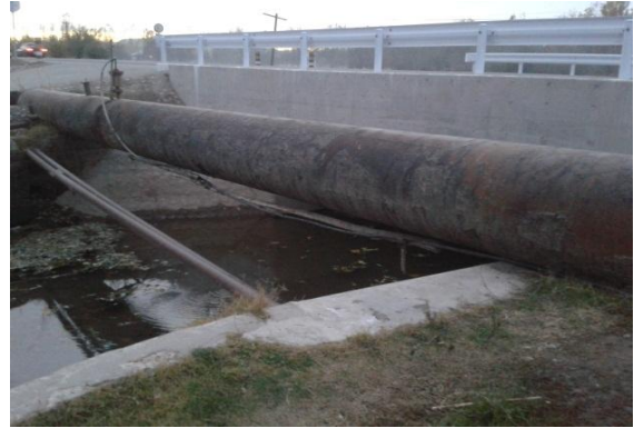
Appearance of culvert 5, at the point 45 km away from Kurgan Tyube (starting point) (at the time of the ex-post evaluation)
