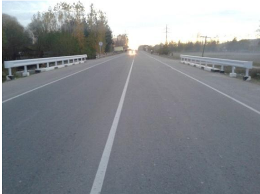
Appearance of the upper part of culvert 5, at the point 45 km away from Kurgan Tyube (starting point) (at the time of the ex-post evaluation)
