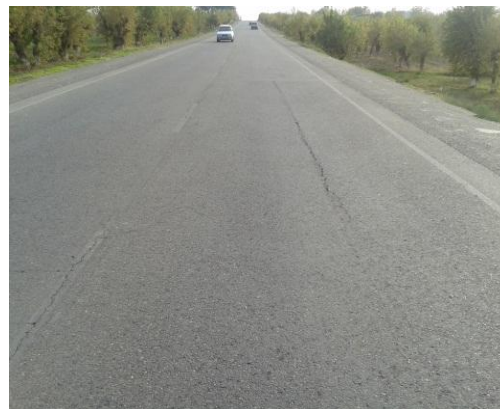
The Road Improved by This Project (At the 52 km point)
