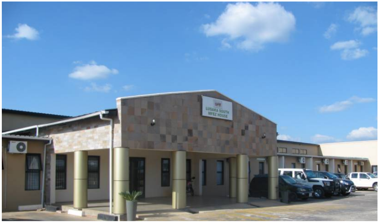
Lusaka South Multi Facility Economic Zone office block
