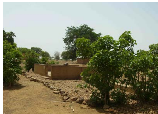
Gravel around the well to avoid a mud puddle and scouring, and hedge to avoid livestock animals (developed by the residents)
