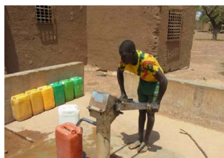
Constructed Deep Well with Hand-pump Facility
