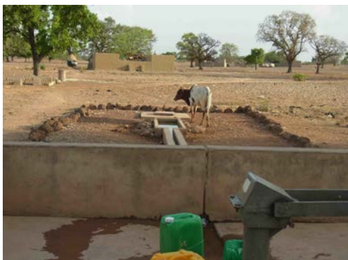
Spilled water from the pump flows to livestock watering hole through drainage
