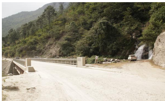
Paving Condition of a Road
