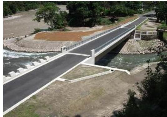
Photograph 2: After Construction Work 16
