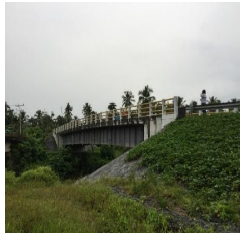
Gido Si'ite Bridge improved by this project
