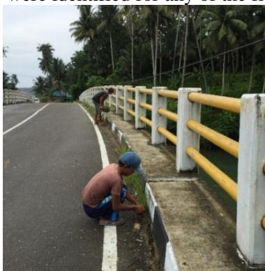
A PPK worker is carrying out weeding work at Sa'au Bridge (at the time of the ex-post evaluation)
