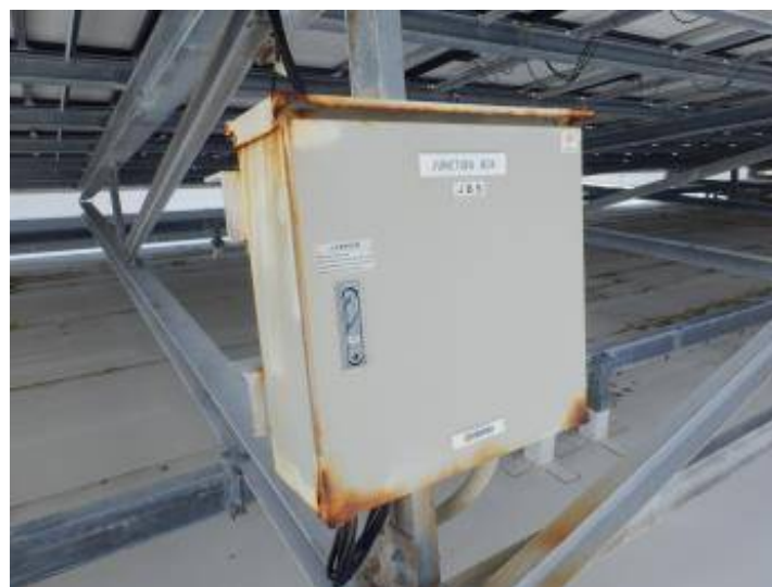
A junction box
