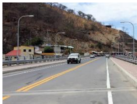
The New Bridge (sight from Ecuadorian side)
