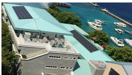
Solar PV Panels on the President Office
