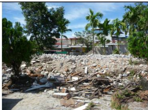
Before the project (December 2009)
