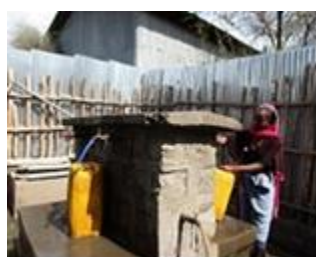
Piped water facility public water faucets
