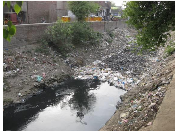
Open Drainage Canal Connecting to the Shad Bagh Pumping Station
