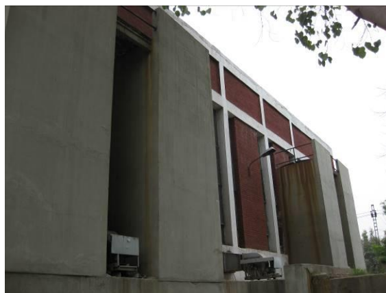
Drainage Basins (Multan Road Pumping Station)
