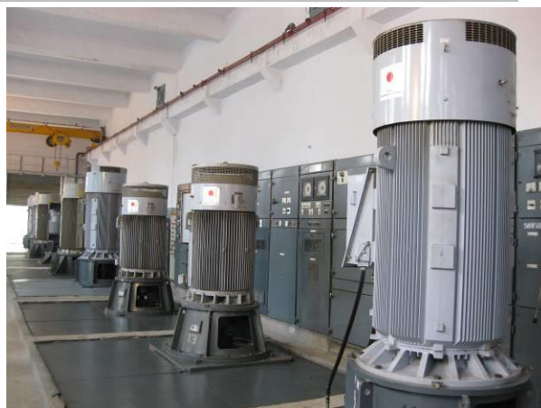
Operation and Electric Room (Gulshan-E-Ravi Pumping Station)
