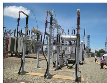
Kiyungi S/S (Reinforcement)
