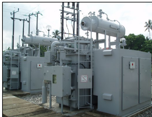
The main transformer of Welezo Substation (33/11kV) newly installed by the project
