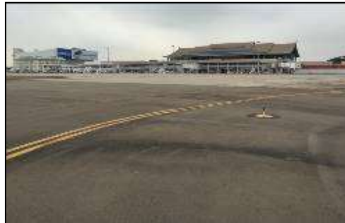
Taxiway Extended (Vientiane International Airport)
