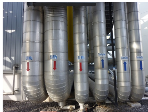
Photo 4: Heat Supplying Pipe
