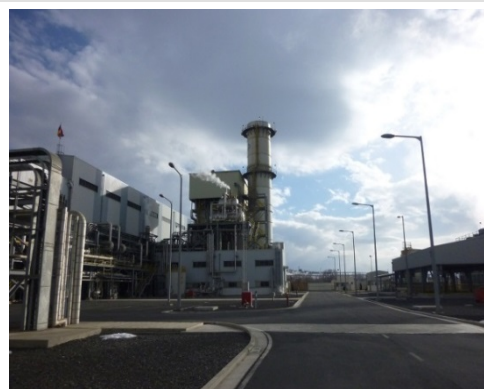
Yerevan Combined Cycle Co-Generation Power Plant
