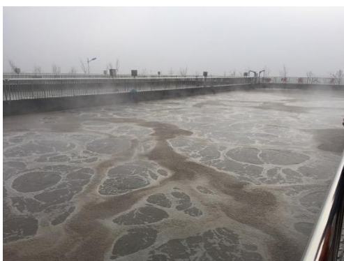
A biological reaction tank at a sewage treatment plant
