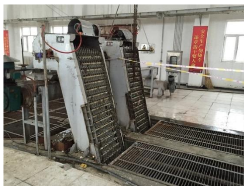
Coarse screens at a sewage treatment plant
