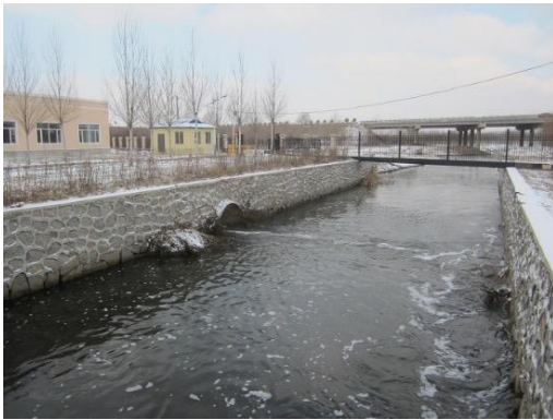
Water discharged from the Pingfang sewage treatment plant
