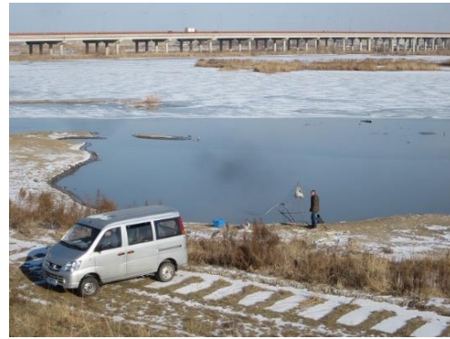
Water discharged from the Songpu sewage treatment plant
