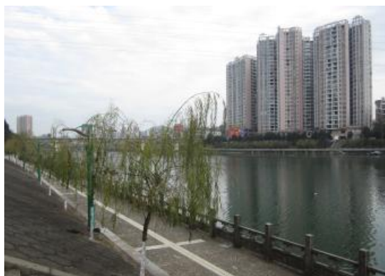
Dike Constructed (in Chibi City)
