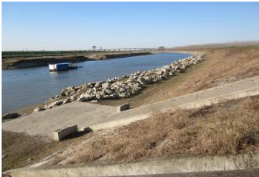
Wave-dissipating concrete blocks (Qianjiang City)
