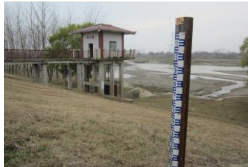
Dike and culvert gate (Xiaogan City)
