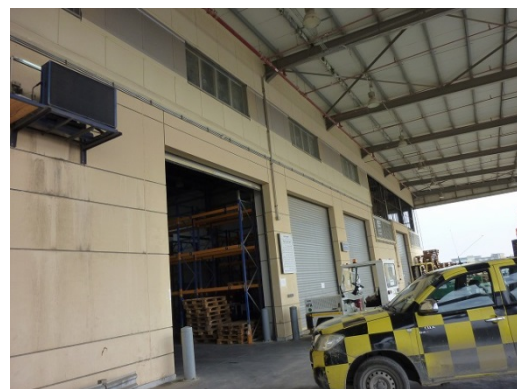
Photo 4: Cargo terminal building built by this project
