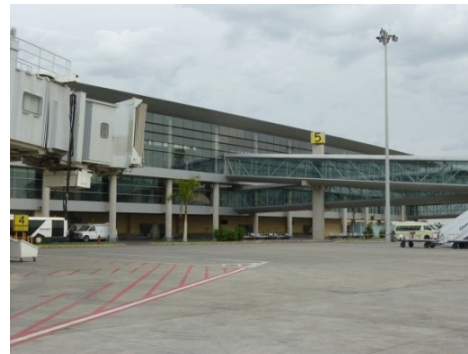
Passenger terminal constructed by this project
