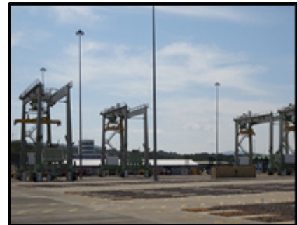
La Union Port: Container terminal, cranes and administration building
