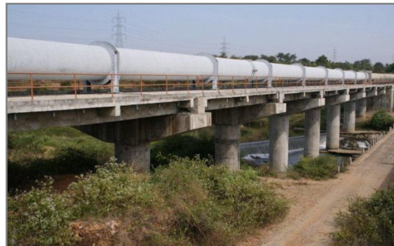
Water Transmission Line to Bangalore City
