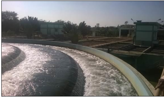
Water Treatment Facility (T.K. Halli)
