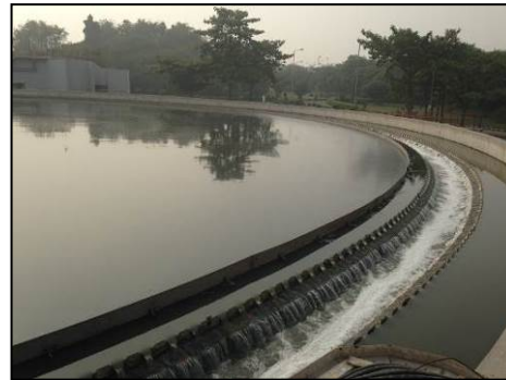
Sewerage Treatment Plant (Okhla)
