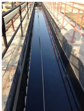
Sewerage Treatment Plant (Western area)
