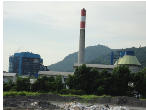
Tarahan Coal Fired Steam Power Plant
