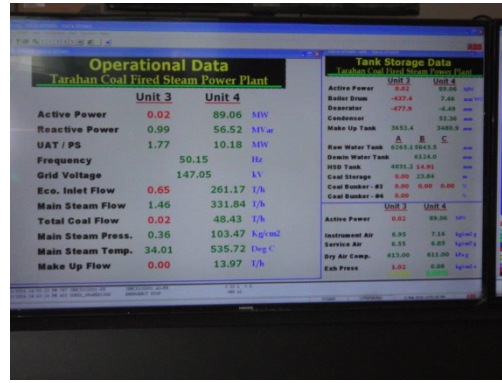
A Scene of the Central Management Room (Display of the PC Monitor)
