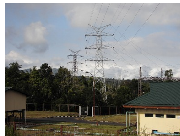
Two Transmission Towers constructed by PLN
