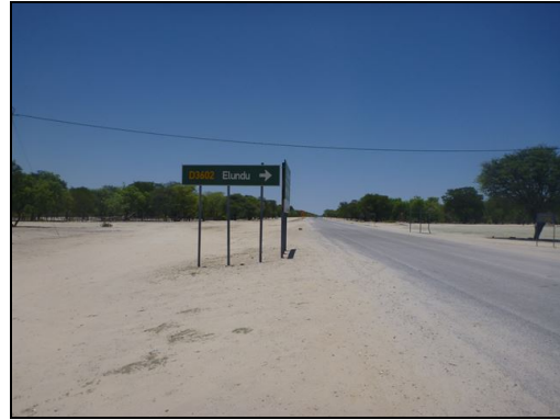
Upgraded Section near Elundu
