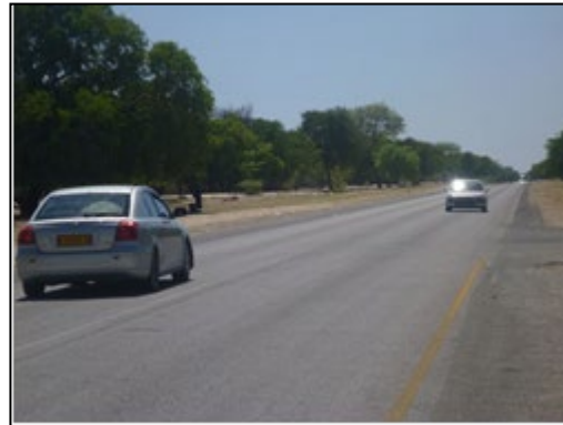
The road improved by this project
