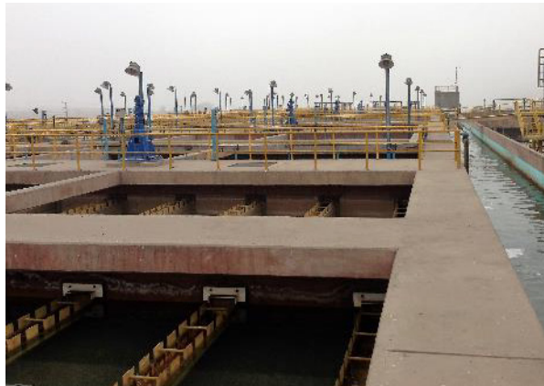
Huachipa Water Treatment Plant
