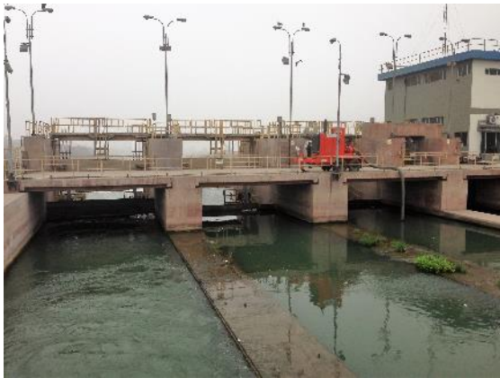
Intake Facility for the Huachipa WTP
