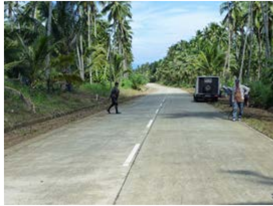
Road Developed by this Project (Kauswagan – Delabayan – Munai Section)
