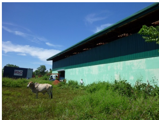
Photo 1: Corn Drying Facility inside MIRAIC (being constructed by the provincial government of Lanao del Norte)
