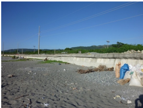
Photo 1: Seawall Protection along the Asian Highway (Ilocos Norte, Region I)
