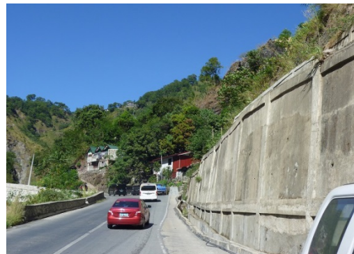
Photo 2: Crib Wall Built along Trunk Road (Abra in CAR)
