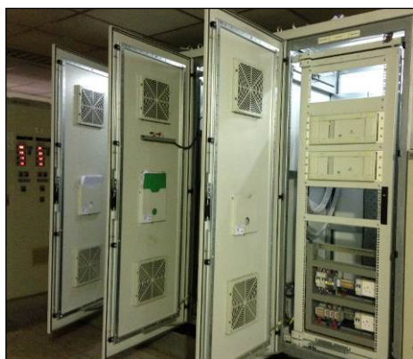
RTU installed (Rawat substation)
