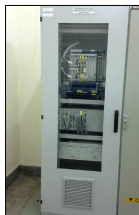
Telecommunication system installed (Substation in Islamabad University)
