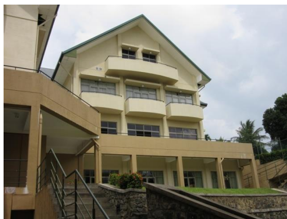
Hotel School Constructed in this Project (In Kandy)
