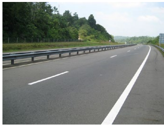
Main Road (Dodangoda-Welipenna section)
