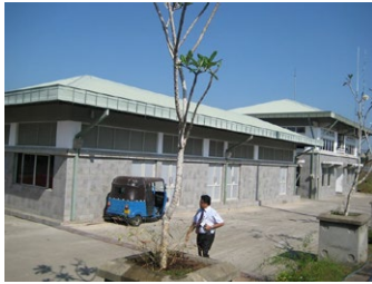
Toll Gate Office (Kottawa)
