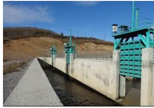
Sile Control Center
