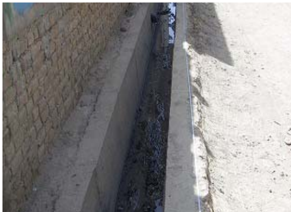
Yakh Kariz: Drainage Construction (At the time of completion)
