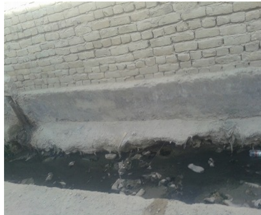
Yakh Kariz: Drainage Construction (At the time of the ex-post evaluation)
