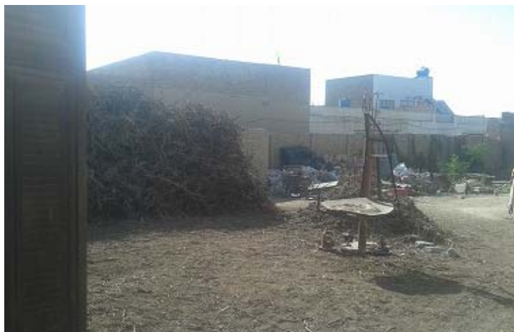
The case where the cow dairy farm was changed into lumber storage place (Yakh Kariz, at the time of the ex-post evaluation)
