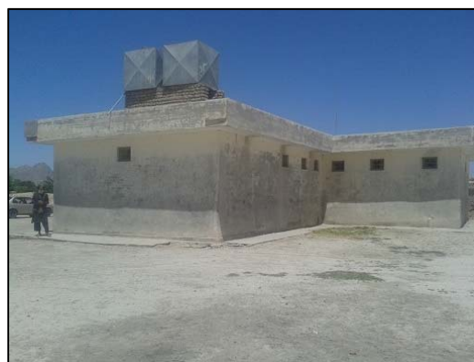
Constructed public bath (at the time of the ex-post evaluation)
