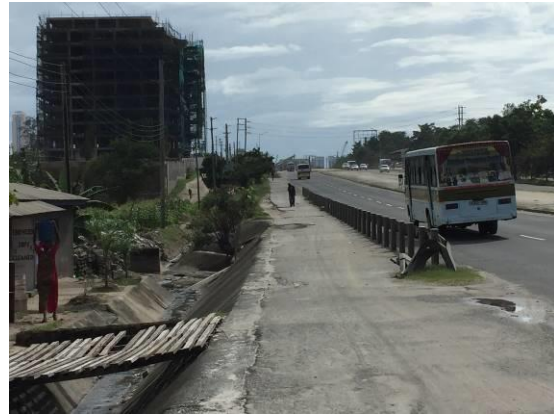
Photo 2: Modern Building under Construction along the Road
