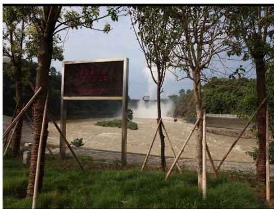
Electronic billboard for warning at Lushui Dam
