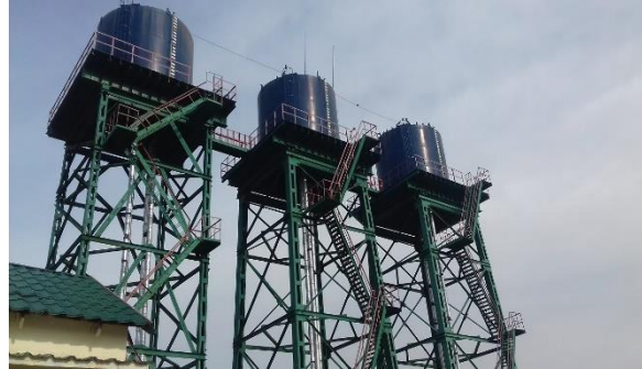
Elevated Water Tank Constructed in This Project
