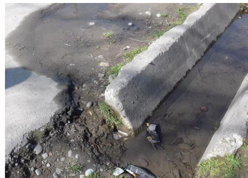
Water Leakage onto Roadways
