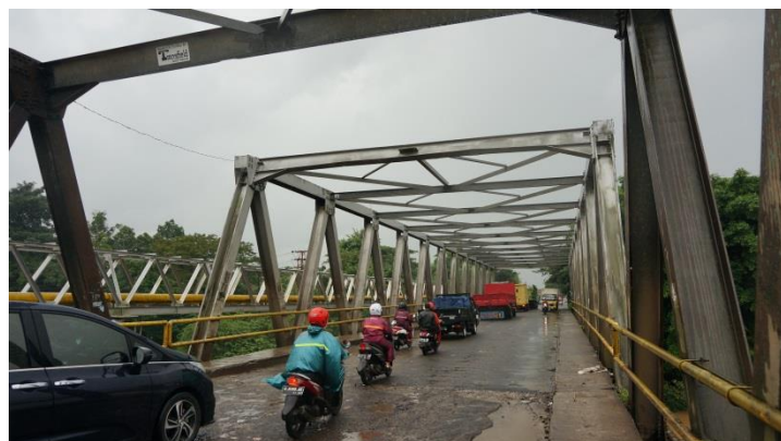
Pilot Project Site for bridge maintenance
