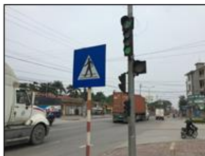
The Installed Traffic Sign and Light
