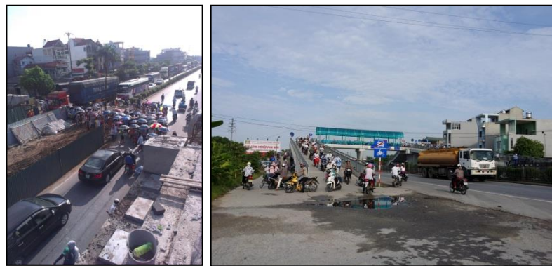
Road Condition Before Installing Overpasses by the Project (left) and After the Project (right)
