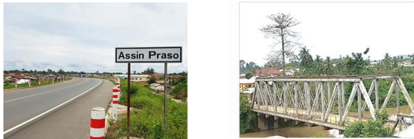
New (left photo) and old (right) Assin Praso Bridge
