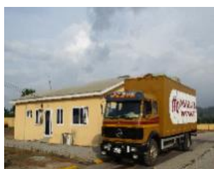
Adansi Asokwa Axle load control station (located 42 km from Assin Praso)
