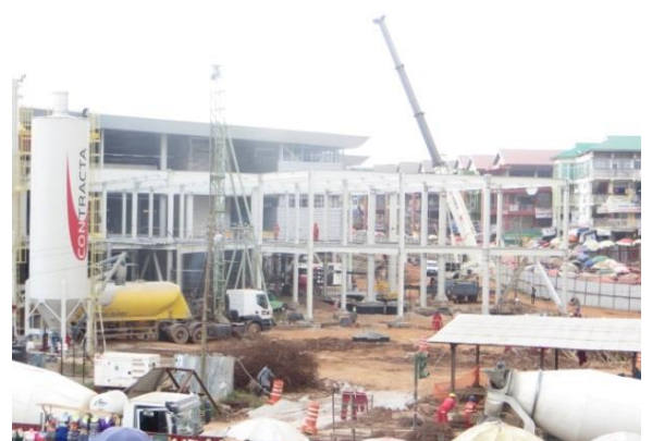
Construction of Kejetia Terminal Complex, Kumasi
