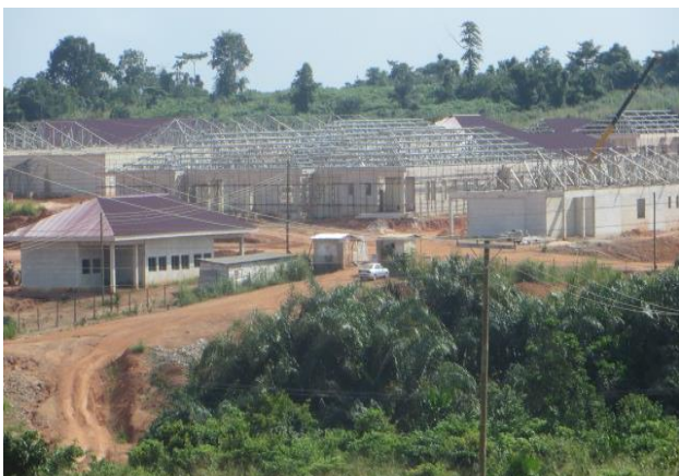
Construction of Regional Hospital, Sewua in the Bosomtwe District
