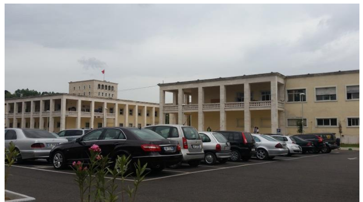
Newly Constructed Parking Facility in Tirana
