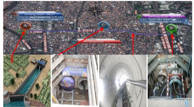
Diversion tunnel from Ciliwung to East Floodway to reduce flood peak discharge by diverting 60 m 3 /s.
