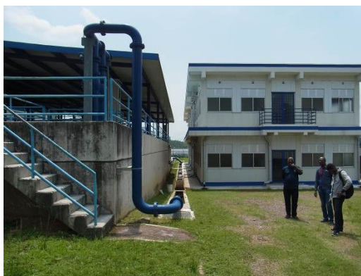
New Water Treatment Plant (extension) and Control Office
