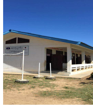
Phonethong primary school built under this project (Champasack, Phonethong)
