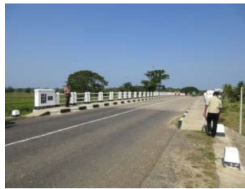
Mundeni Bridge (No.2 Bridge) after reconstruction
