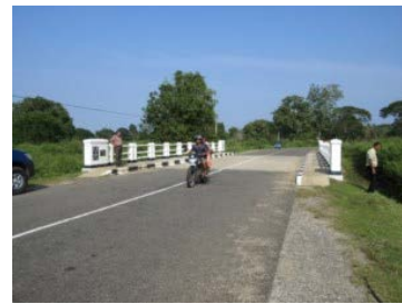
Pulavady Bridge (No.3 Bridge) after reconstruction
