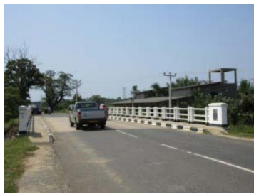
Mahaoya Athuganga Bridge (No.1 Bridge) after reconstruction
