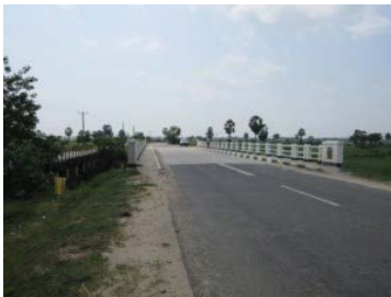
Chenkalady Bridge (No.4 Bridge) after reconstruction
