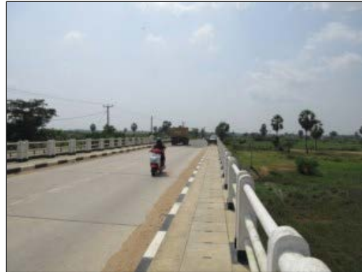
Vehicles passing over the Chenkalady Bridge (Bridge No.4) after reconstruction.
