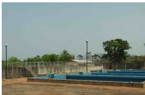
Constructed water treatment plant
