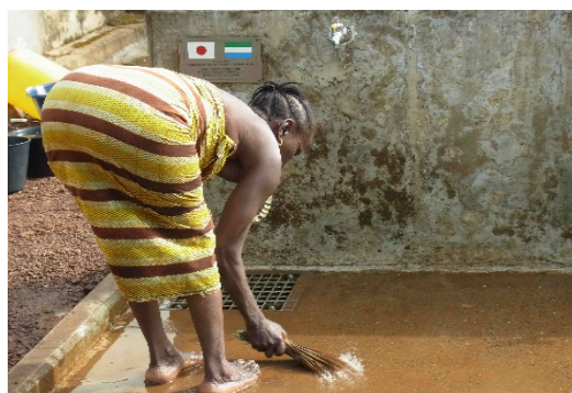
Cleaning public water taps by pump attendant
